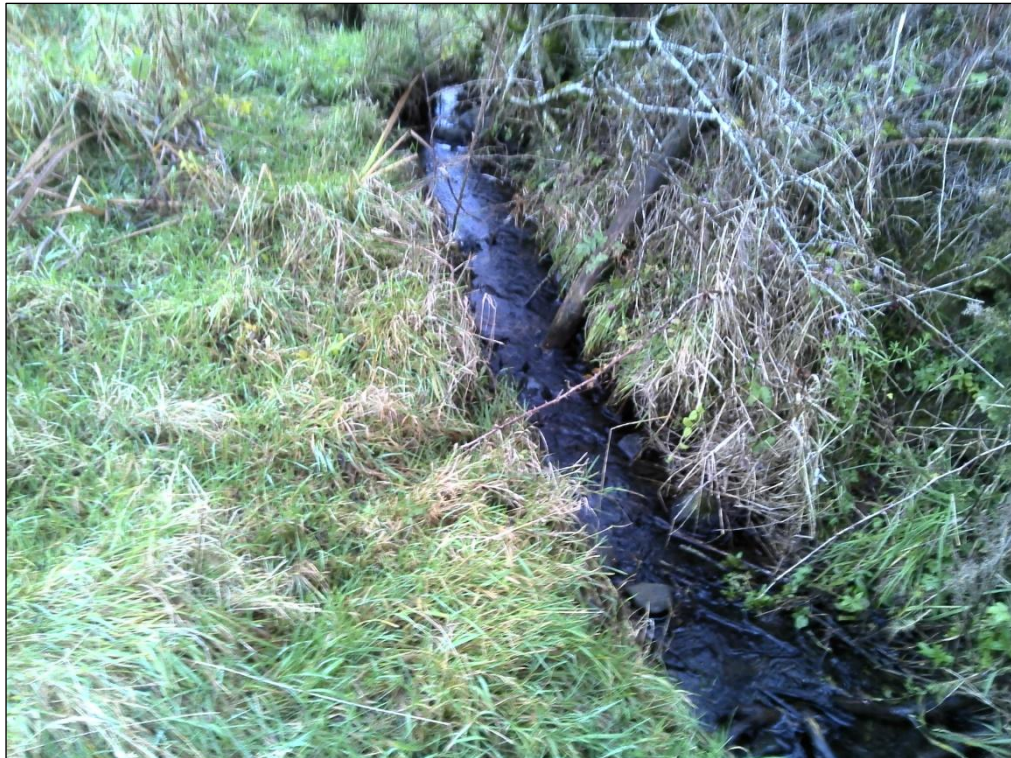
Plate 2.9. Watercourse at chainage 22+175.
